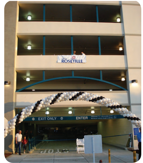
Parking structures are a key element to promoting single trip parking
