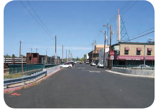
Existing Atlantic Street between Taylor and Vernon Streets
